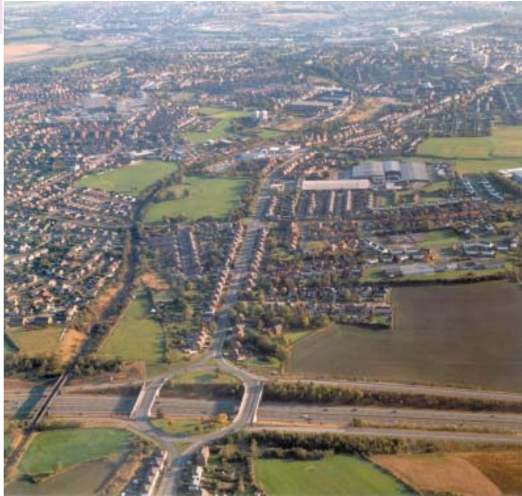
Junction 37 of the M1, with Barnsley Town Centre in the background (top right)
